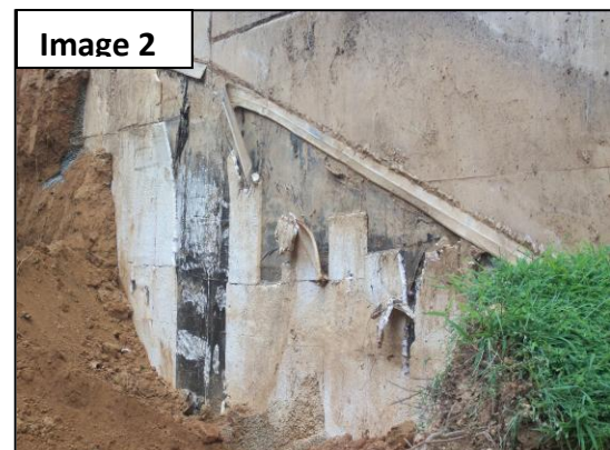
Existing Foundation Waterproofing
